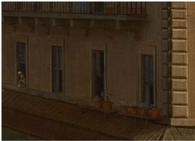
Fig. 10 Detail of the first floor of the building in the immediate foreground on the right
